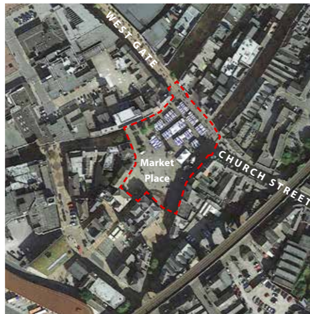
Figure 1.20: Aerial view of existing
