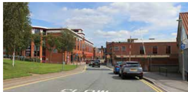
Figure 1.27: Photo of the existing site and surrounding streets
