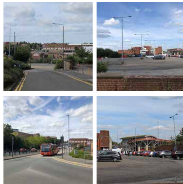
Figure 1.65: Photos of the existing site and surrounding streets
