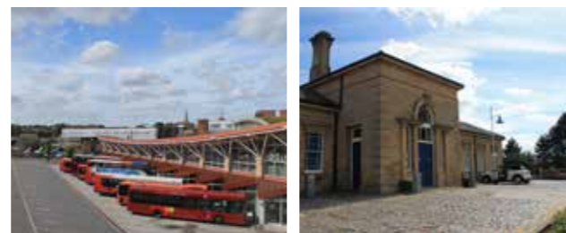
Figure 1.73: Photos of the existing site and surrounding streets
