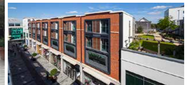
Figure 1.85: Parkway, Newbury created a new retail street connected to the existing high street with residential above and behind creating new public and private amenity spaces
