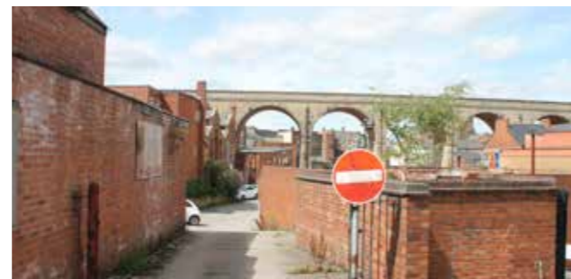
Figure 1.32: Photos of the existing site and surrounding streets
