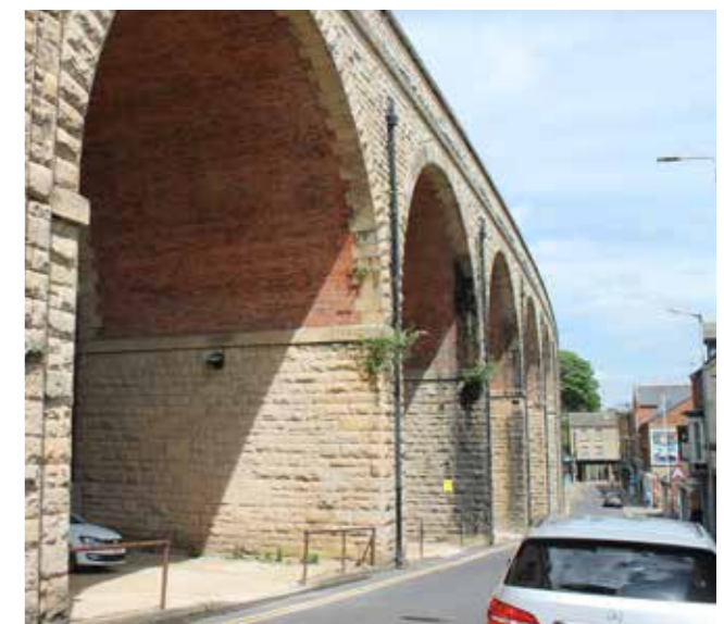
Figure 1.50: Photos of the viaduct today
