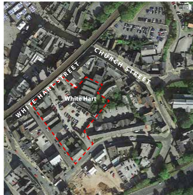
Figure 1.31: Aerial view of existing
