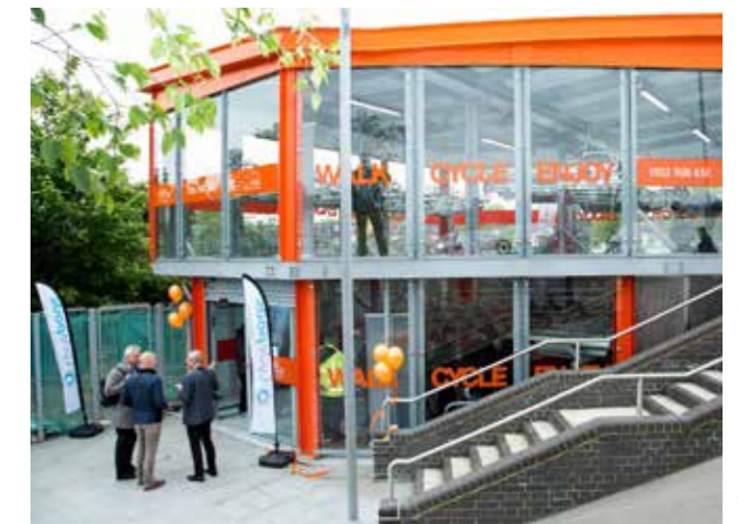
New cycle hubs have been installed at key stations in Waltham Forest. These have CCTV, key fob entry, lighting, tyre pumps and tiered cycle storage. These secure facilities make it easier for people commuting or shopping locally to travel by bike
