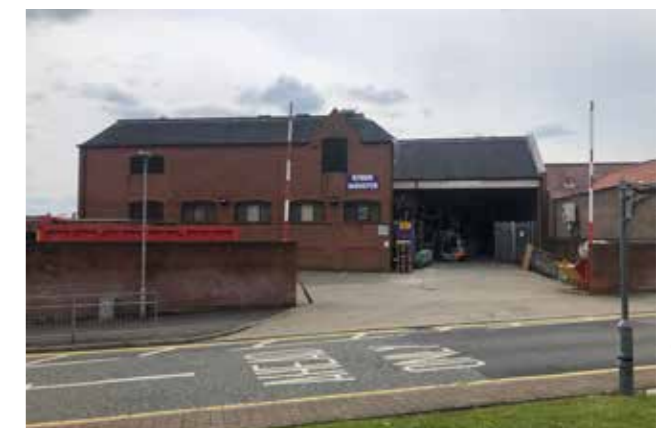
Figure 1.19: Clumber Street service yard frontage
