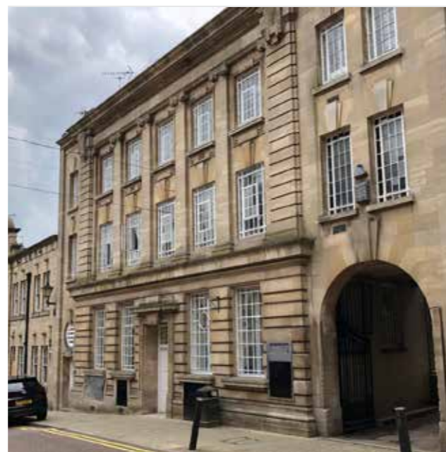
Figure 1.46: Photos of the existing building
