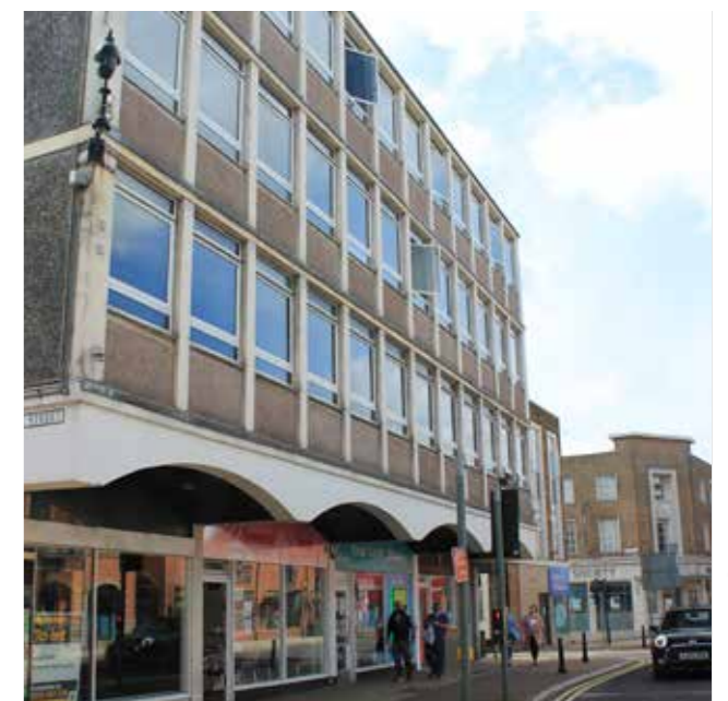
Figure 1.30: Photos of the existing building
