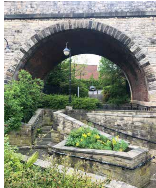
Figure 1.49: Photos of the viaduct
