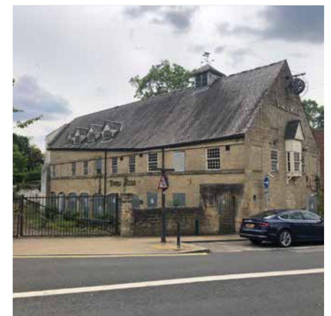
Figure 1.48: Photos of the existing building
