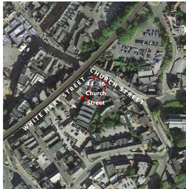
Figure 1.45: Aerial view of existing
